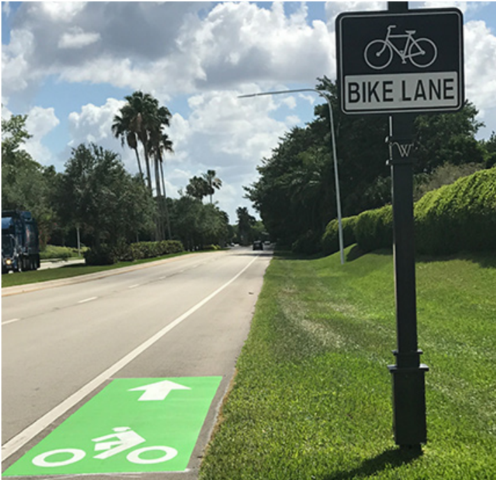
Figure 3.3: Weston bike lane street lane marking and signage.
